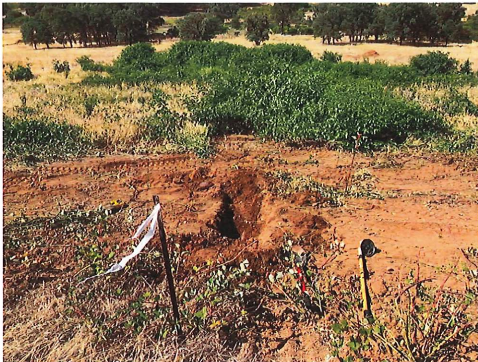
Photo No. 3 View looking directly downslope (southwest) from the top of Field A. Excavation LF4 is in the foreground (photo date 8/7/2020).
