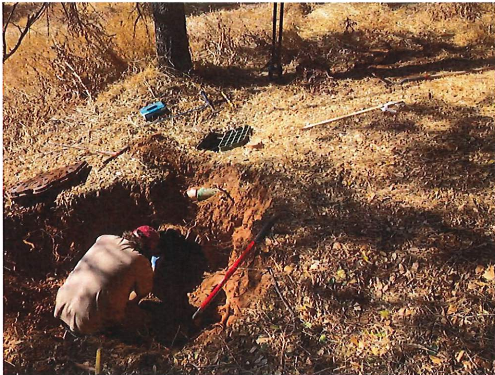
Photo No. 9 Northeast end of Field B, Row 2 infiltrator exposed in excavation LF3. View is looking to the southwest (photo date 8/7/2020).
