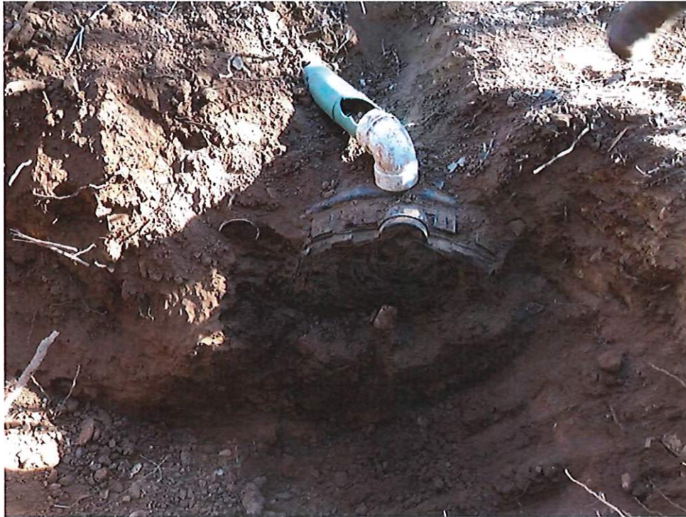
Photo No. 7 Southwest end of Field B, Row 4 infiltrator exposed in excavation LF2. (photo date 8/7/2020).
