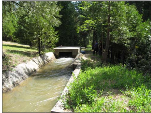
Photo 5 – Outlet Structure at Buffalo Hill
