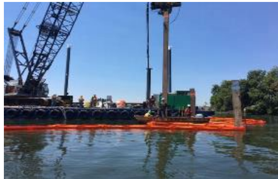
Smith Canal Flood Gate Project Construction
