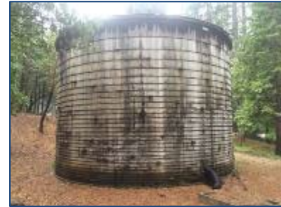
Amador Water Agency Water Tank
