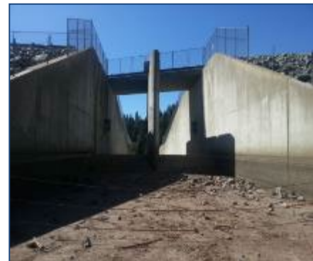
Sugar Pine Dam Spillway
