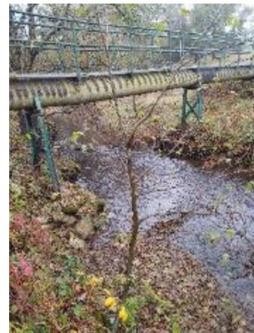
Doty North Canal Project Site
