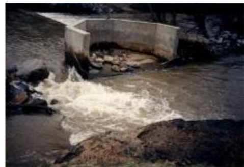
Hemphill Diversion Structure Project Site
