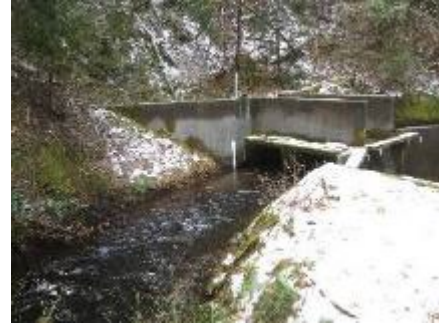
Six Stream Gages and Mutton Canyon Creek Project Site
