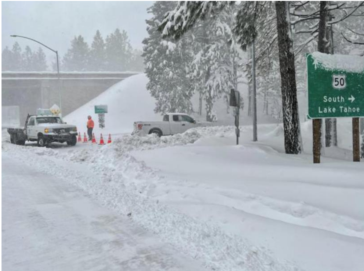
Figure 4-41 2023 Snowfall Impacting Roads Near South Lake Tahoe
