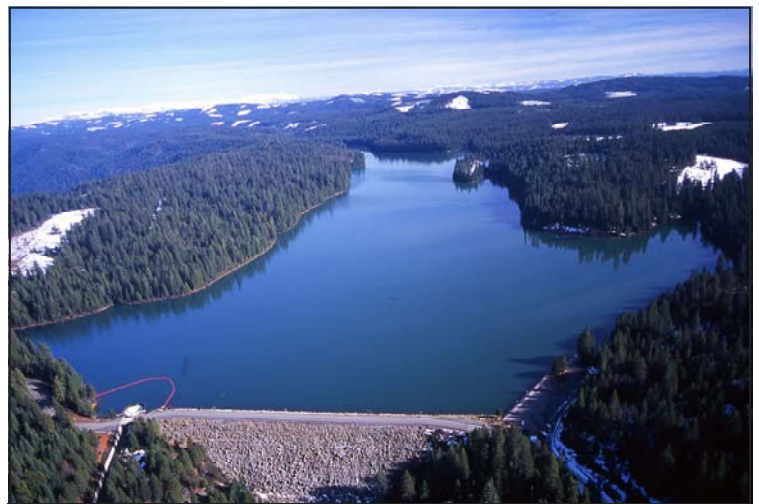
The District applied for water rights licensing of Stumpy Meadows in 2010. Stumpy stores 20,000 acre feet of water and is the source of the water for the Divide communities.
