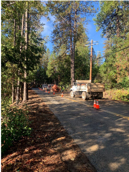
Main Break Repair – 50 Labor Hours | Dump Truck, Vac Trailer, Service Trucks, Hand Tools
