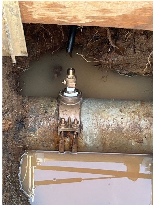
Lateral Break Repair – 36 Labor Hours | Dump Truck, Vac Trailer, Service Trucks, Hand Tools
