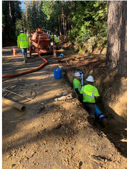
Main Break Repair – 50 Labor Hours | Dump Truck, Vac Trailer, Service Trucks, Hand Tools
