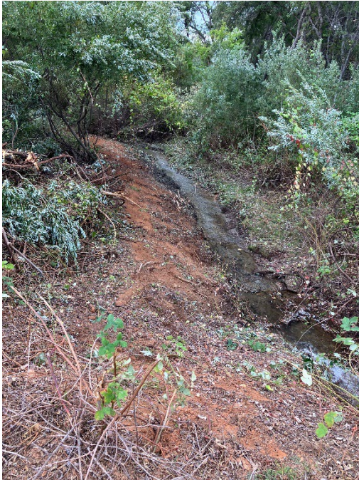
Vegetation Clearing Task – ~500 Feet | 23 Labor Hours | Trimmers, Brush Cutters, Mini-Excavator
