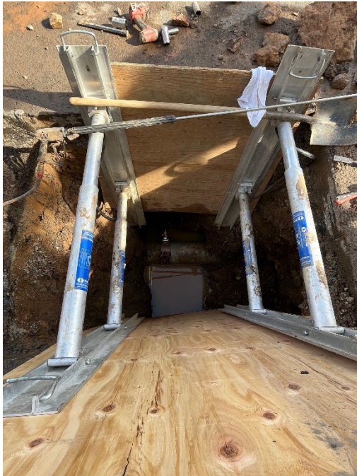
Lateral Break Repair – 36 Labor Hours | Dump Truck, Vac Trailer, Service Trucks, Hand Tools
