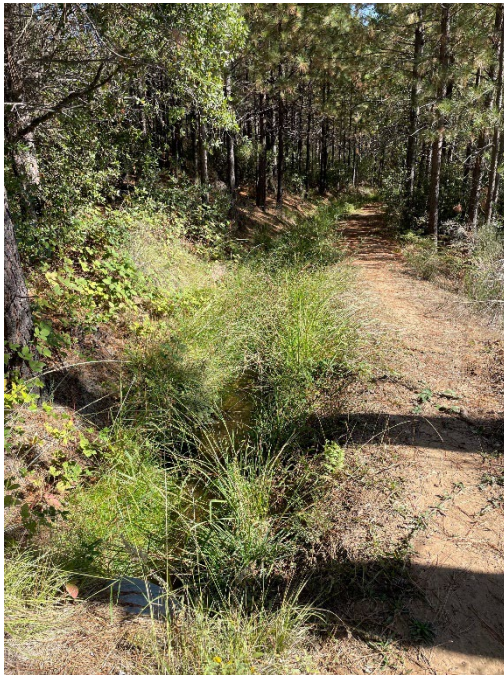
Vegetation Clearing Task – ~250 Feet | 8 Labor Hours | Trimmers, Brush Cutters
