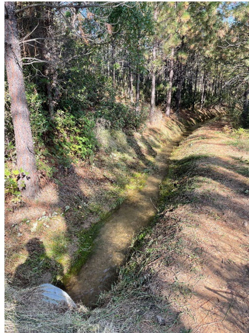
Vegetation Clearing Task – ~250 Feet | 8 Labor Hours | Trimmers, Brush Cutters
