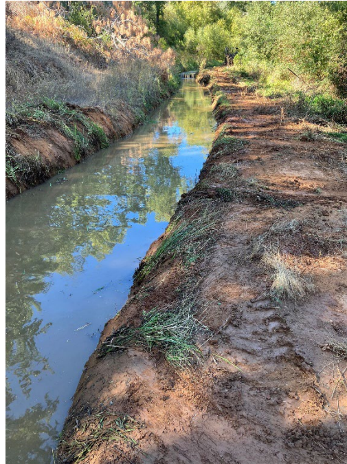
Vegetation Clearing Task – ~500 Feet | 23 Labor Hours | Trimmers, Brush Cutters, Mini-Excavator
