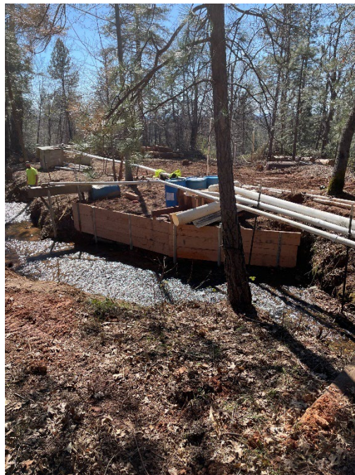
Tree Removal/Irrigation Service Repair/Crib Wall Repair – 87 Labor Hours | Excavator, Service/Dump Truck, Hand Tools, Materials
