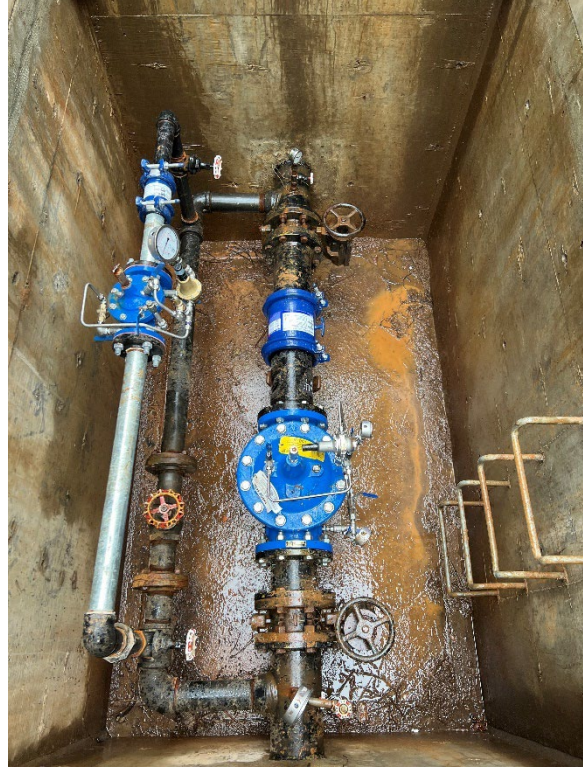
Pressure Reducing Valve Replacement – 18 Labor Hours | Excavator, Service Truck | PRV, Fittings
