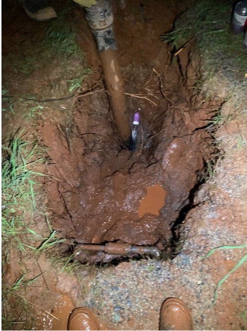
Service Line Repair – 21 Labor Hours | Excavator, Vacuum Trailer, Service/Dump Truck, Hand Tools, Light Trailer
