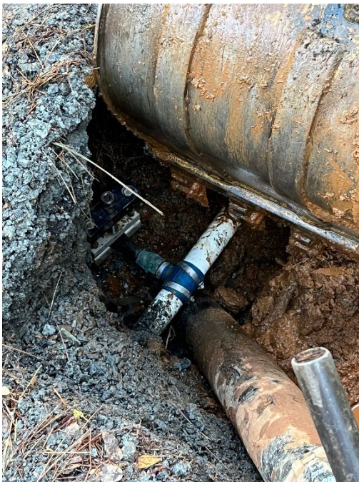
Service Line Repair – 20 Labor Hours | Excavator, Dump/Utility Truck, Vacuum Trailer, Parts
