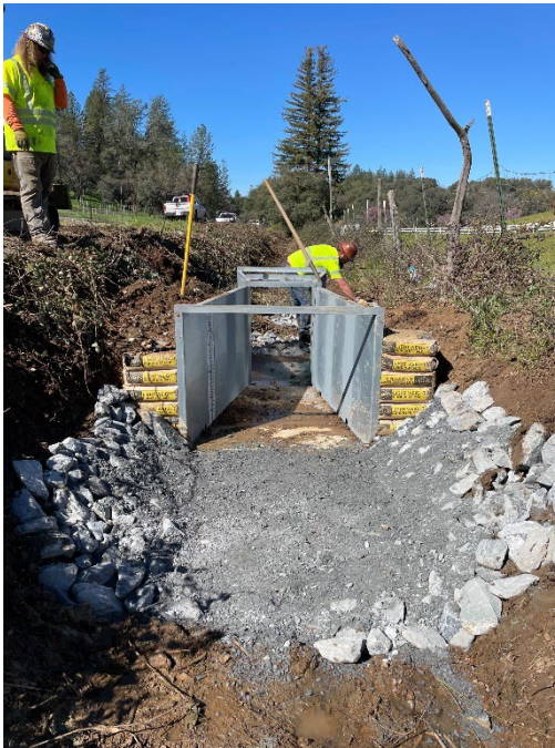
Raw Water Flume Installation – 86 Labor Hours | Service Truck, Dump Truck, Excavator
