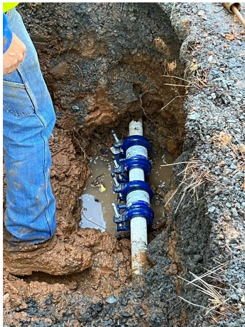
Service Line Repair – 20 Labor Hours | Excavator, Dump/Utility Truck, Vacuum Trailer, Parts
