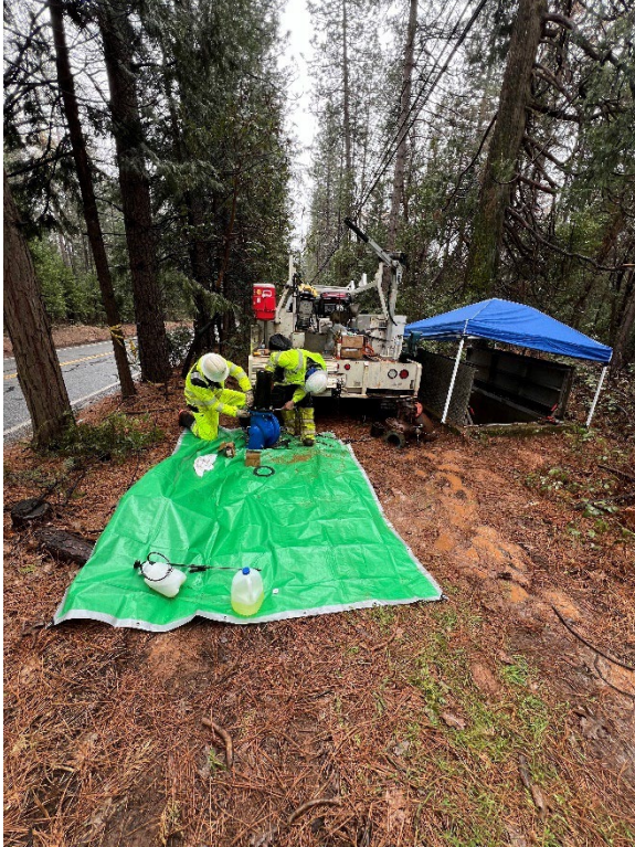
Pressure Reducing Valve Replacement – 18 Labor Hours | Excavator, Service Truck | PRV, Fittings
