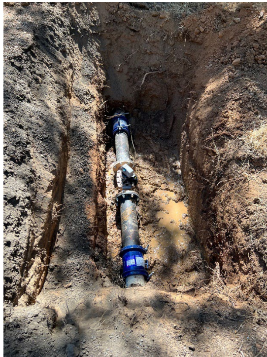
Garden Valley Master Meter Install – 48 Labor Hours | Service Trucks, Excavator, Dump Truck, Vacuum Trailer
