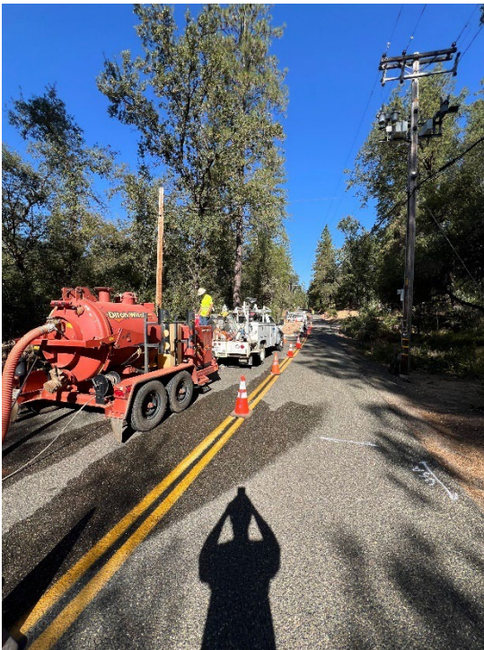
Garden Valley Master Meter Install – 48 Labor Hours | Service Trucks, Excavator, Dump Truck, Vacuum Trailer
