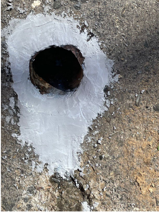
Stumpy Spillway Underdrain Deflectors/Concrete Repair – 12 Labor Hours | Service Truck
