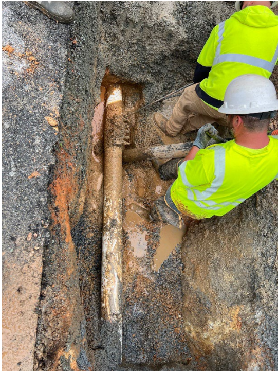
Water Main Break – 35 Labor Hours | Service Trucks, Excavators, Dump Trucks, Vacuum Trailer
