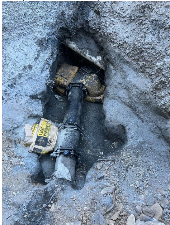
Hydrant Lateral Repair – 72 Labor Hours | Service Trucks, Excavators, Dump Trucks, Vacuum Trailer
