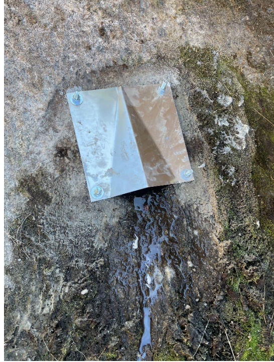
Stumpy Spillway Underdrain Deflectors/Concrete Repair – 12 Labor Hours | Service Truck
