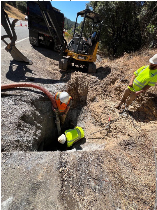
Hydrant Lateral Repair – 72 Labor Hours | Service Trucks, Excavators, Dump Trucks, Vacuum Trailer
