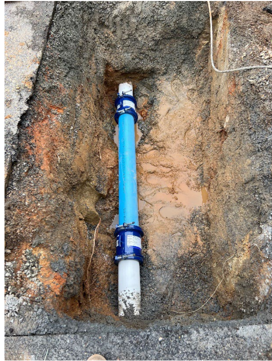
Water Main Break – 35 Labor Hours | Service Trucks, Excavators, Dump Trucks, Vacuum Trailer
