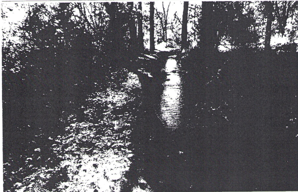
LN 06-11-6:28: View S40W, Georgetown Divide Ditch within project area (gunite-lined).
