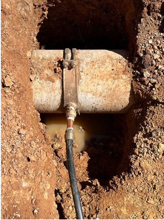
Lateral Repair – 79 Labor Hours | Excavator, Loader, Service Trucks, Dump Trucks
