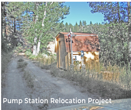
Funding Acquisition for Pump Station Relocation Project
