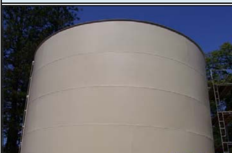
Black Oak Mine Tank Exterior
