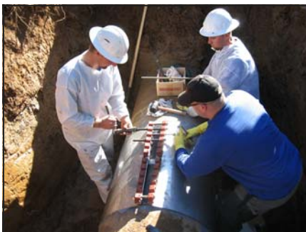
Bottom Left: Crews make a repair band to fix a raw water pipe near ALT Water Treatment Plant. Jacob Walsh (L), Chris Barbour (R back) and Matt Sampson (R front) are the crew members.
