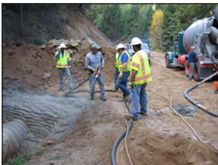
Top Left: Crews repair 300 feet of pipe in an area that is geologically unstable. They shotcrete the head wall to prevent water seeping into the piped section.
