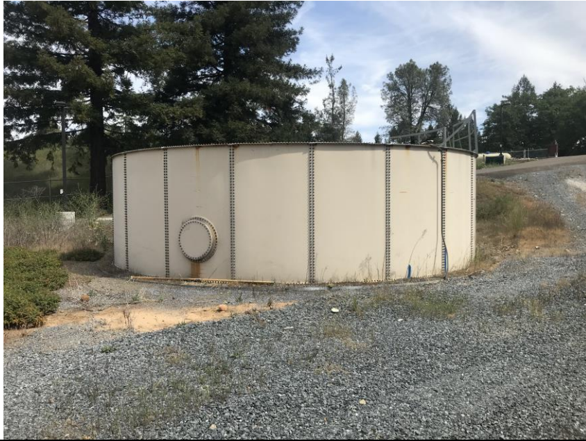
View of water storage tank.
