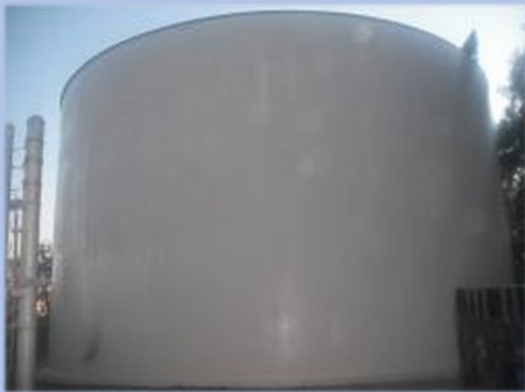
Spanish Dry Diggins Storage Tank
