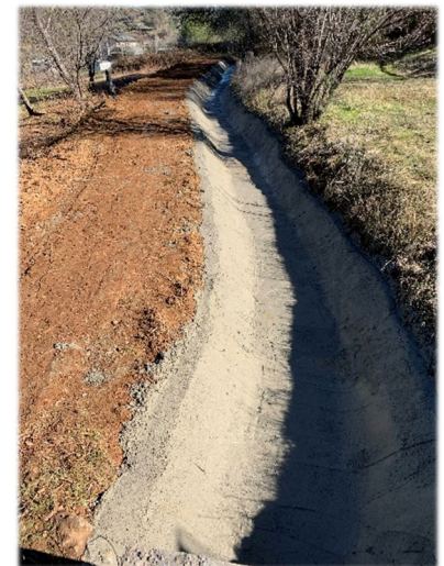
Lined Section of Canal
