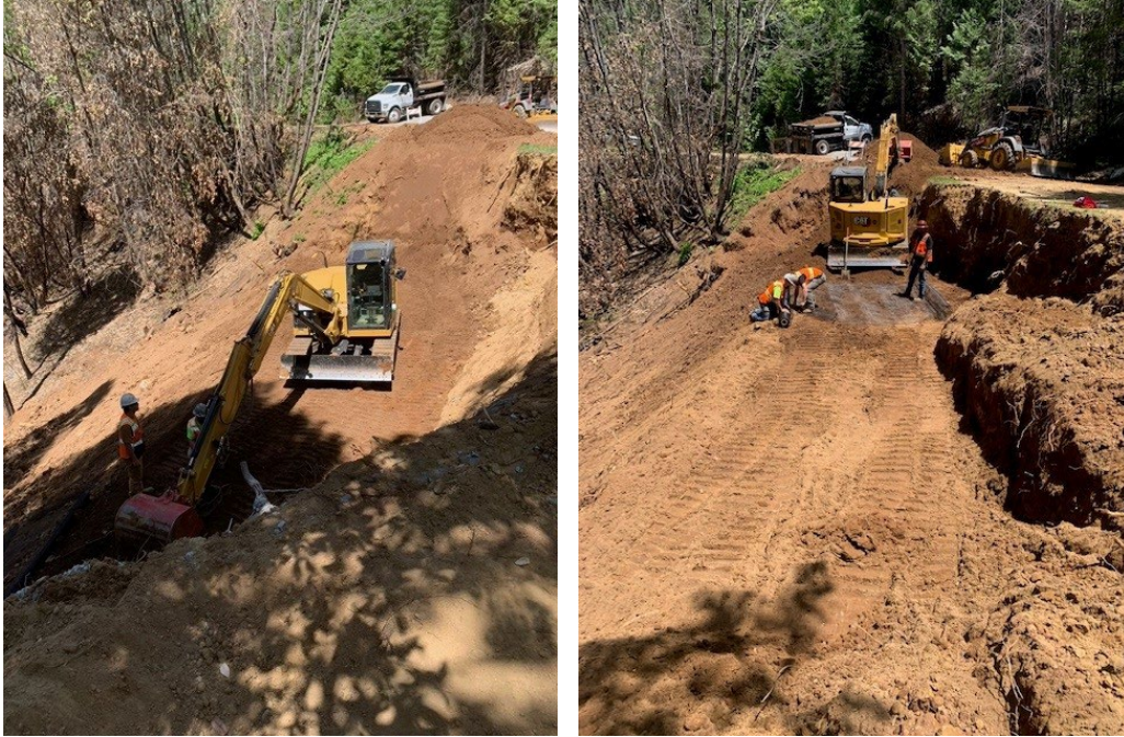
Benching and Geogrid Installation
