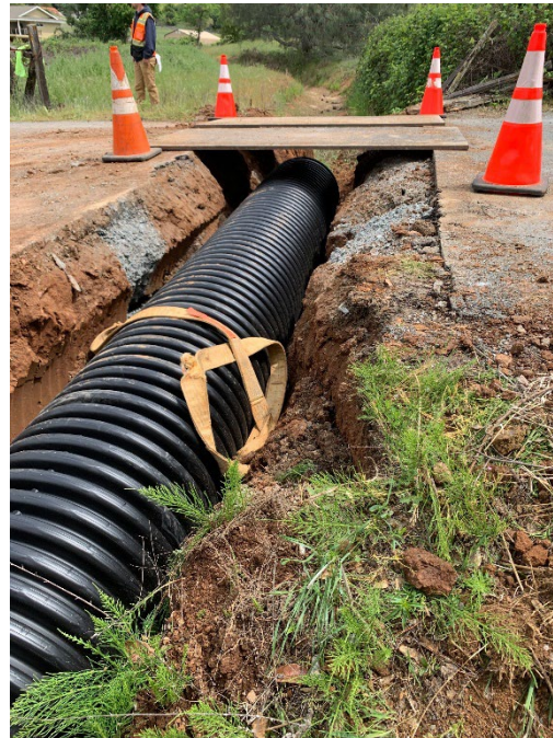
Meter/Antenna Installation | Culvert Installation
