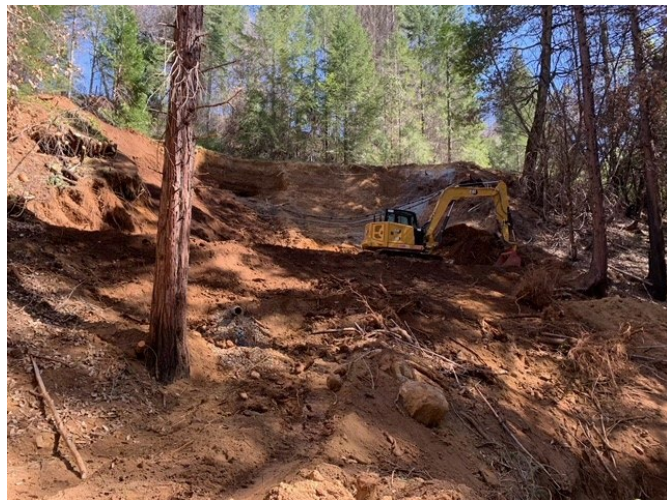
Soil Delivery and Benching
