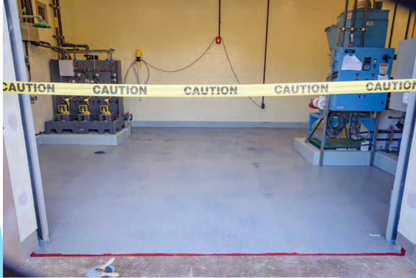
Repainted Floor of Chemical Storage Room
