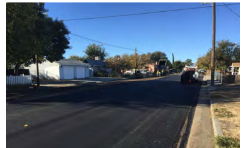
2017 Pavement Repair Project
