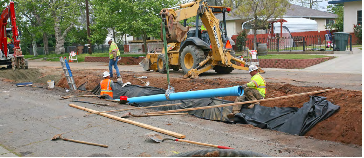
Downtown Waterline and Street Replacement Project – City of Lincoln
