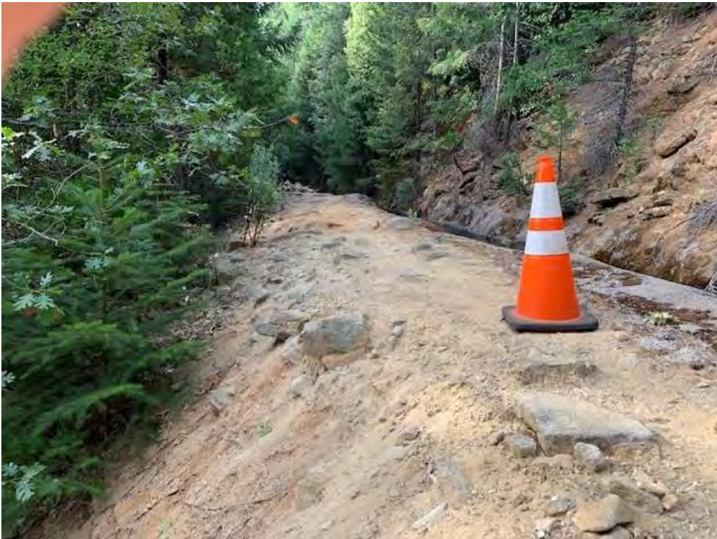
Picture 2 – Downslope of ditch bank looking upstream.
