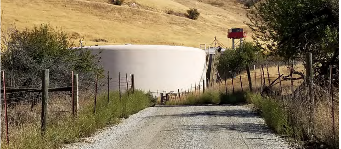
Cement Hill Pipeline Replacement Project – Suisun Solano Water Authority
