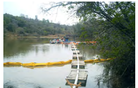
Clover Valley Reservoir Desilting and Reservoir Supply Pipeline– PCWA
