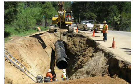
Gold Run Pipeline, Phase IV – PCWA
