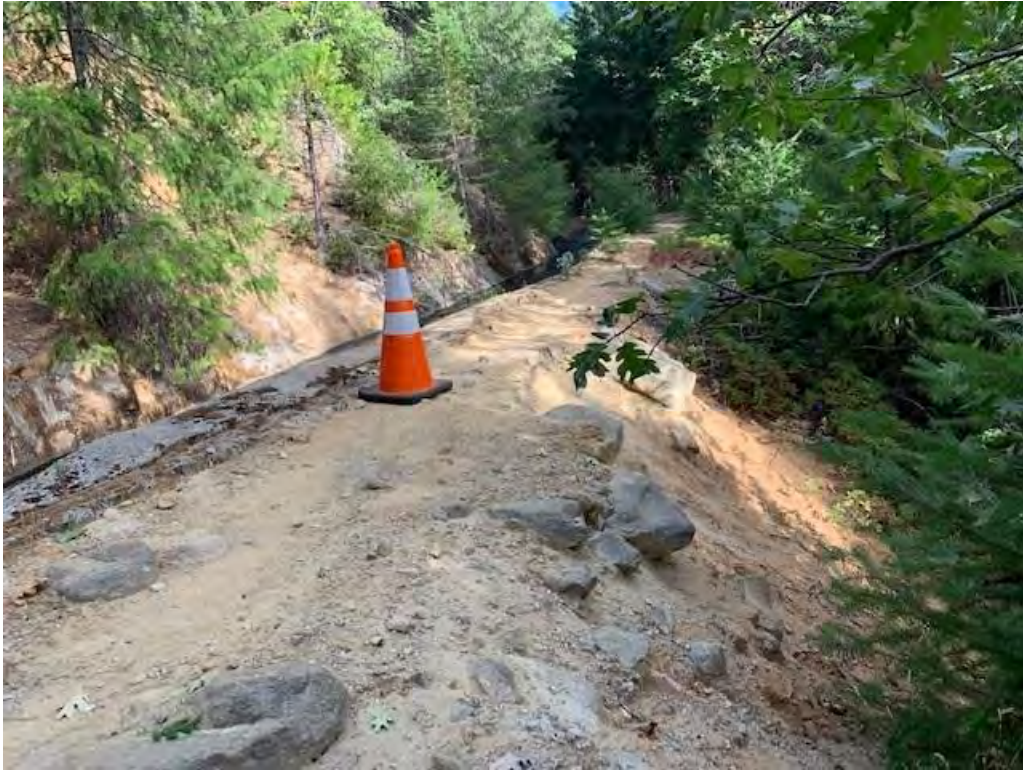
Picture 1 – Downslope of ditch bank looking downstream.
