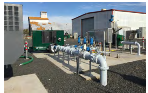
Wastewater Treatment Plant Improvements
