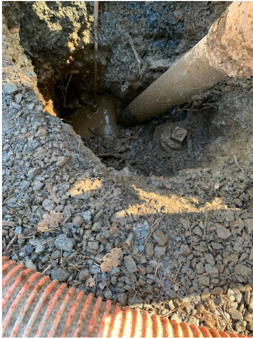
Main Break Repair – 15 Labor Hours | Dump Truck, Vac Trailer, Service Trucks, Hand Tools
