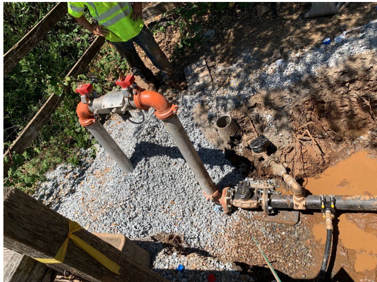
4-Inch Meter Installation – 44 Labor Hours | Dump Truck, Vac Trailer, Excavator, Service Trucks, Hand Tools
