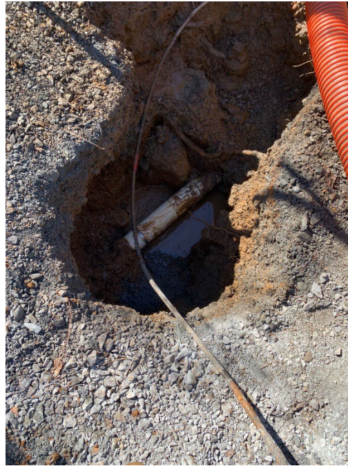
Main Break Repair – 15 Labor Hours | Dump Truck, Vac Trailer, Service Trucks, Hand Tools
