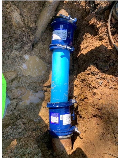
Main Break Repair – 36 Labor Hours | Dump Truck, Vac Trailer, Service Trucks, Hand Tools
