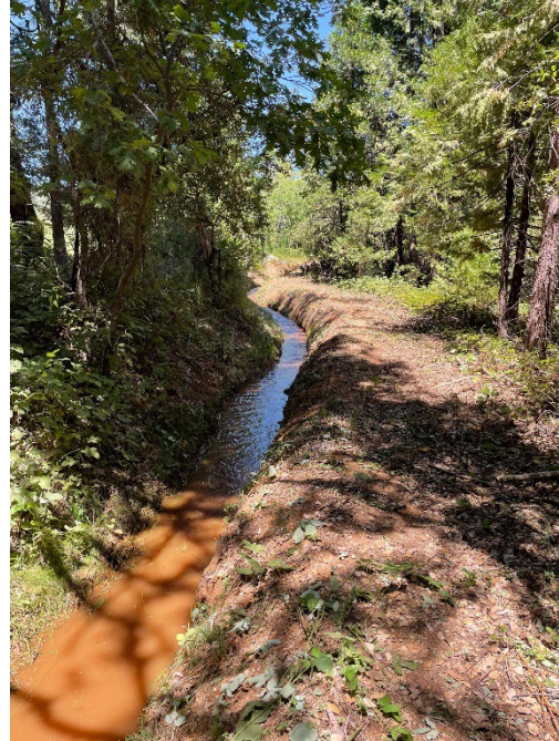
Vegetation Clearing Task – ~350 Feet | 22 Labor Hours | Trimmers, Brush Cutters
