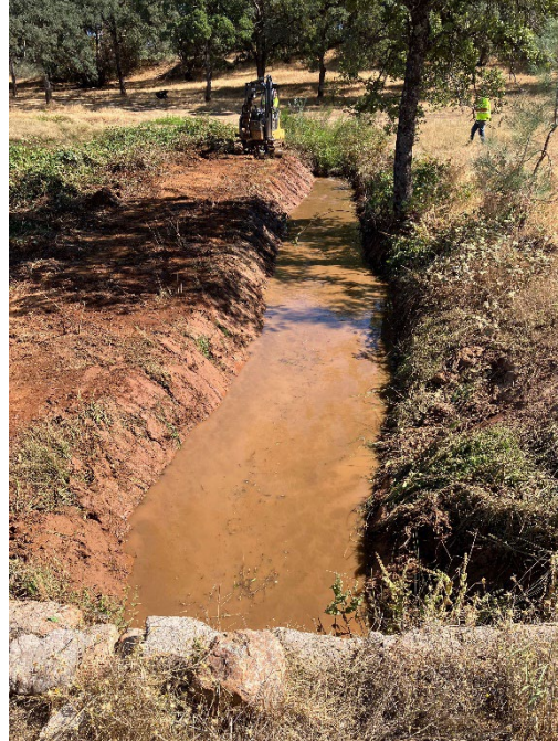
Vegetation Clearing Task – ~450 Feet | 19 Labor Hours | Trimmers, Brush Cutters, Mini-Excavator
