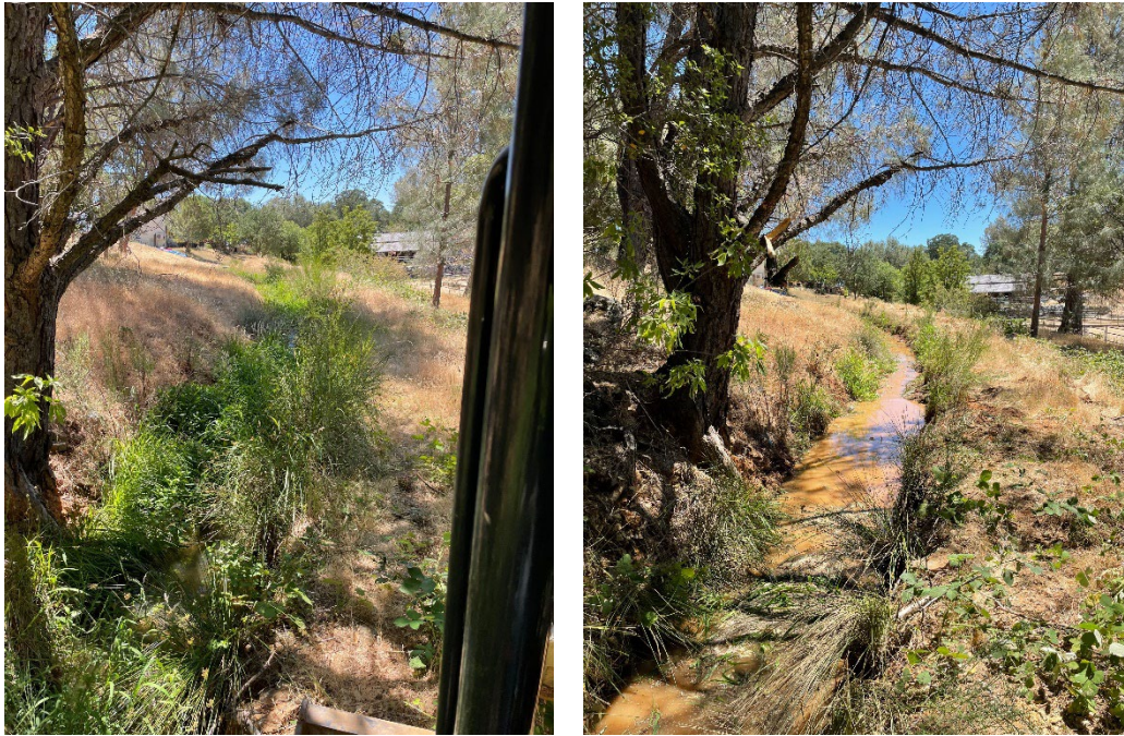
Ditch Cleaning – ~360 Feet | 16 Labor Hours | Mini-Excavator, Hand Tools
