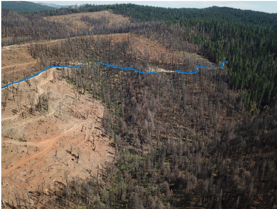
Sierra Pacific Industries Operations – Up Stream Structure #3
