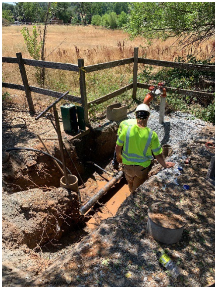
4-Inch Meter Installation – 44 Labor Hours | Dump Truck, Vac Trailer, Excavator, Service Trucks, Hand Tools
