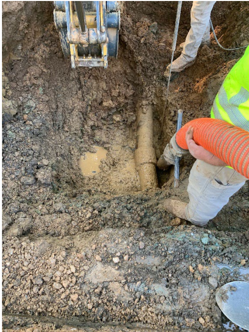
Main Break Repair – 36 Labor Hours | Dump Truck, Vac Trailer, Service Trucks, Hand Tools
