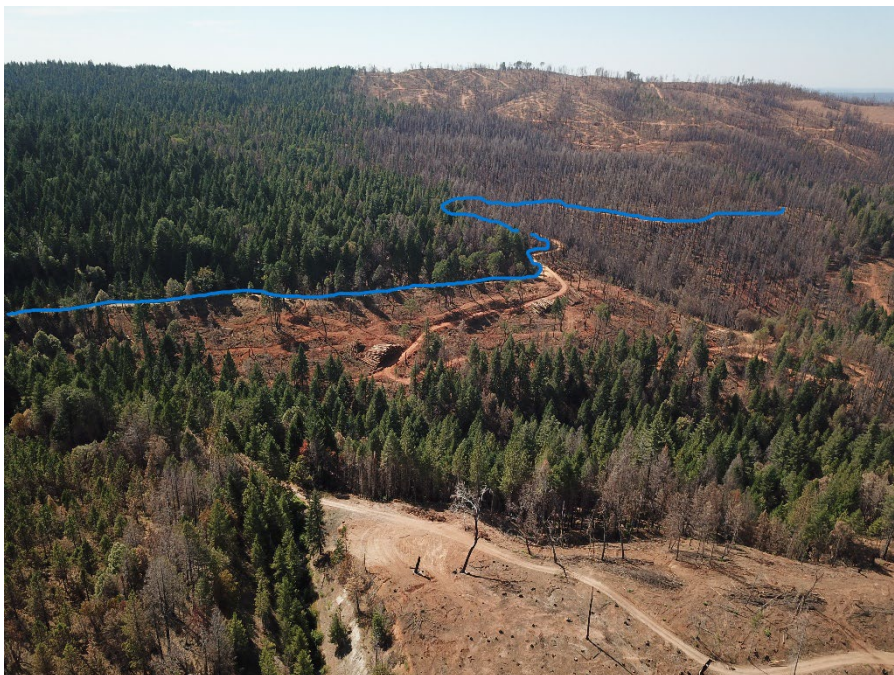
Sierra Pacific Industries Operations – Down Stream Structure #5
