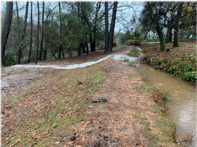
Ditch Storm Surge
