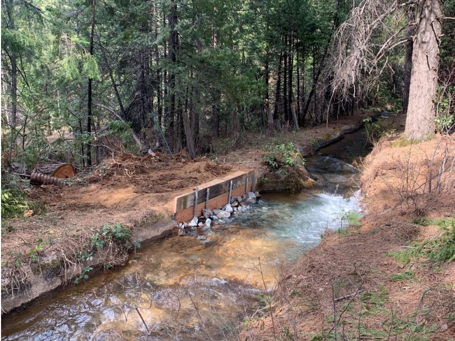
Upper ditch tree damage crib wall repair
