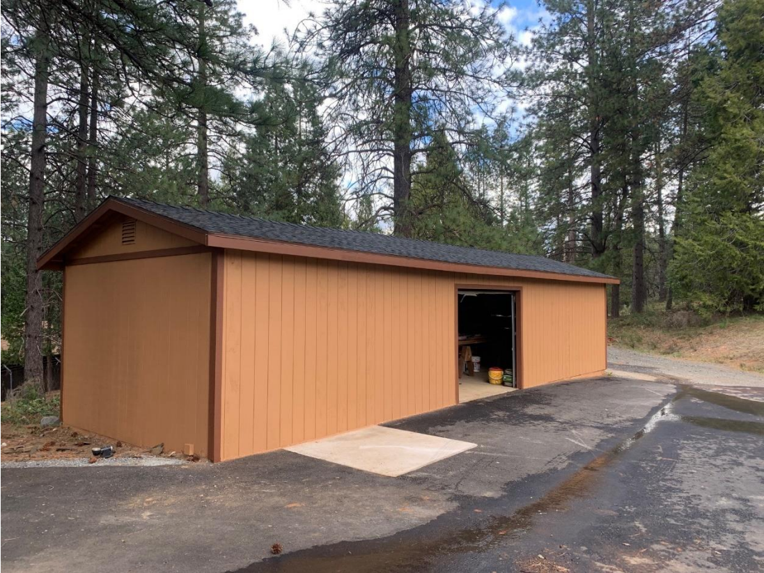
Office Shed Rebuild
