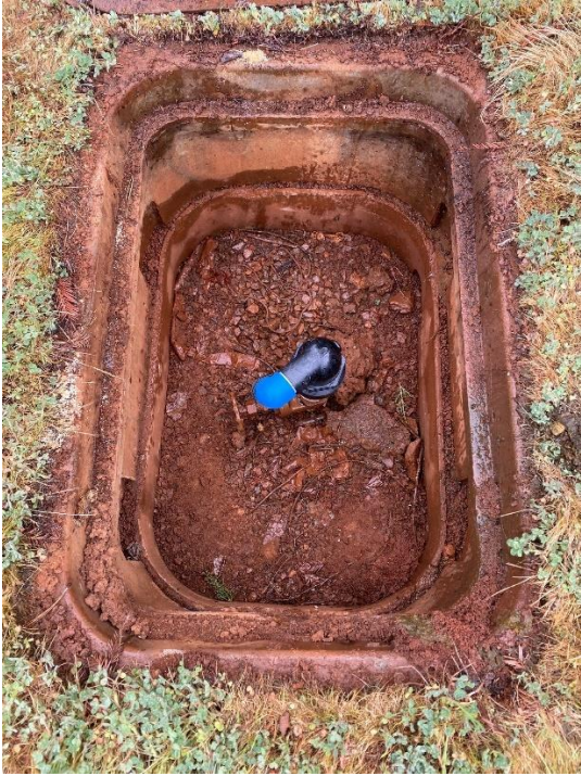
Air Relief Valve Replacement – New vs. Old
