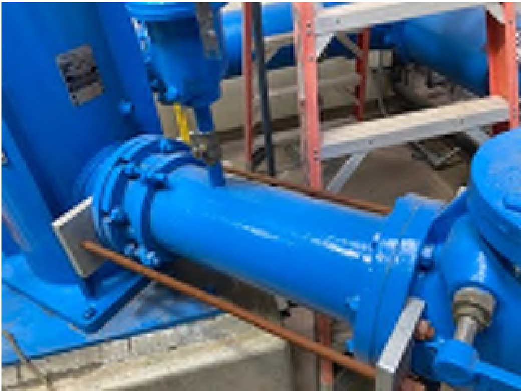
Figure 2 - 8" Pump Discharge with Increaser
