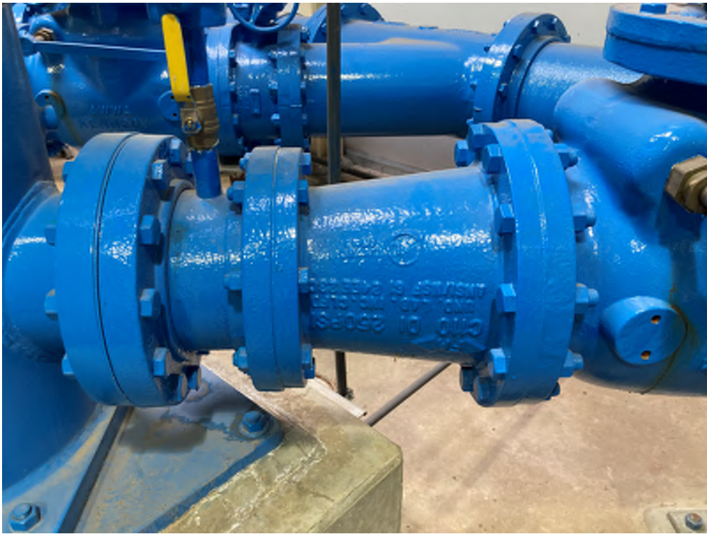
Figure 1 - 10" Pump Discharge with Increaser
