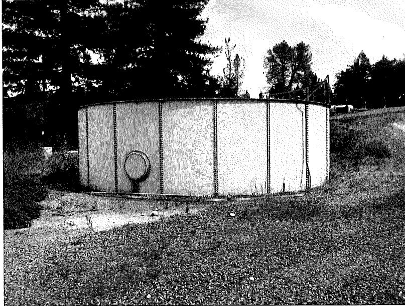
View of water storage tank.
