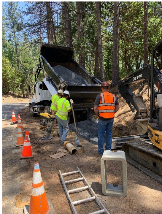
Master Meter Installation (Reservoir Road) – 35 Labor Hours | Utility Trucks, Excavator, Material, Vac Trailer, Dump Trucks
