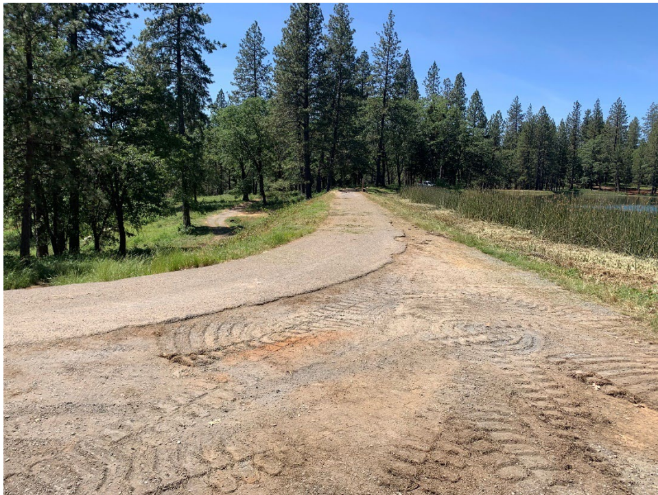
Vegetation Clearing – 8 Labor Hours | Excavator, Masticator, Service Truck
