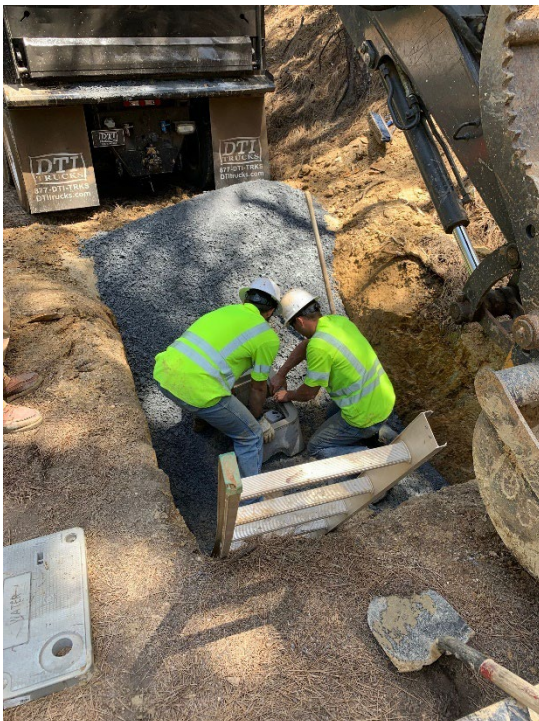
Master Meter Installation (Reservoir Road) – 35 Labor Hours | Utility Trucks, Excavator, Material, Vac Trailer, Dump Trucks
