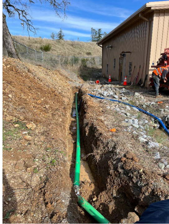
Raw Water Building Drain Repair – 40 Labor Hours | Excavator, Service Trucks, Ditch Witch, Dump Truck
