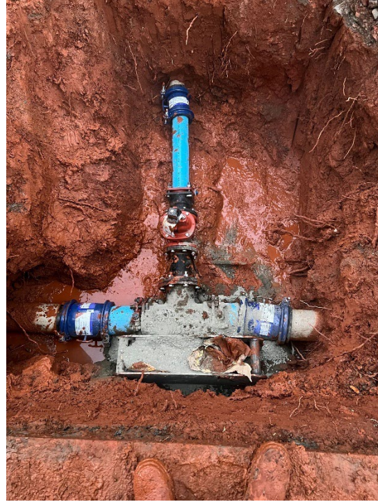
Main Line Repair – 95 Labor Hours | Excavator, Service Trucks, Ditch Witch, Dump Truck
