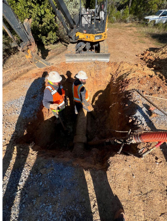
Georgetown Master Meter Installation – 35 Labor Hours | Excavator, Service Trucks, Ditch Witch, Dump Truck
