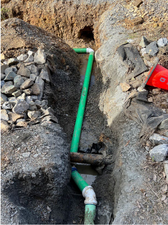
Raw Water Building Drain Repair – 40 Labor Hours | Excavator, Service Trucks, Ditch Witch, Dump Truck
