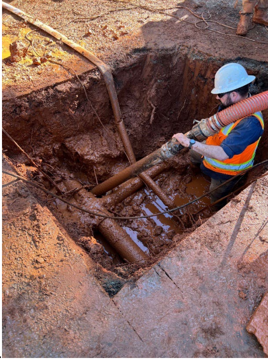
Main Line Repair – 95 Labor Hours | Excavator, Service Trucks, Ditch Witch, Dump Truck
