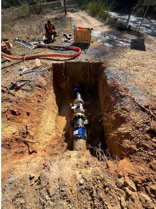
Georgetown Master Meter Installation – 35 Labor Hours | Excavator, Service Trucks, Ditch Witch, Dump Truck
