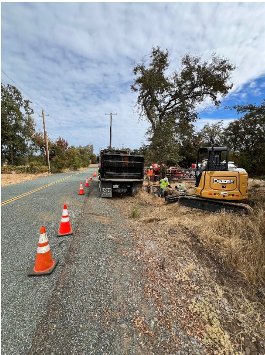
Pilot Hill Master Meter Install – 29 Labor Hours | Service Trucks, Dump, Excavator, Vac Trailer
