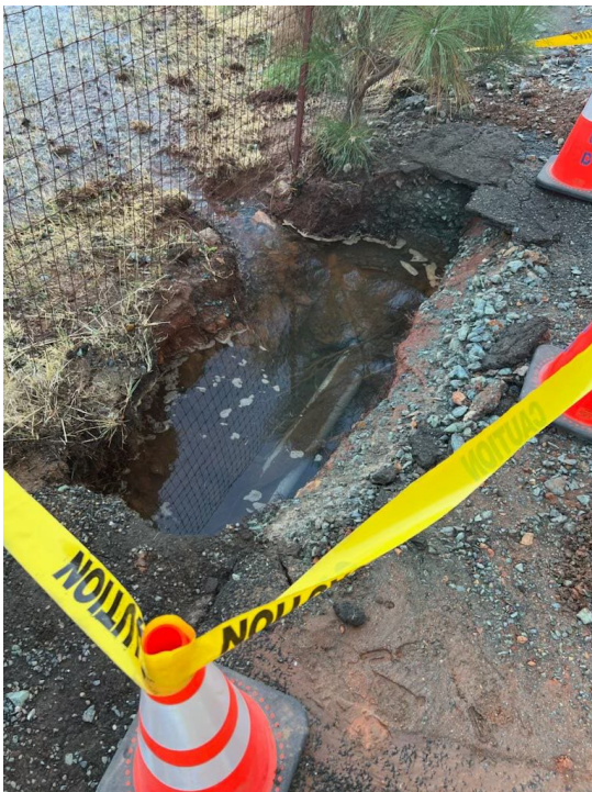
Main Break – 47 Labor Hours | Excavator, Service Truck, Ditch Witch, Loader, Sampling, Dump Truck
