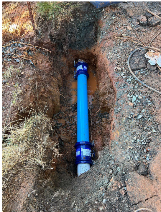
Main Break – 47 Labor Hours | Excavator, Service Truck, Ditch Witch, Loader, Sampling, Dump Truck
