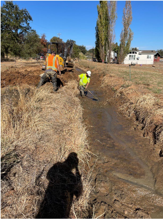
Canal Lining Preparation (Cool) – 76 Labor Hours | Service Trucks, Dump, Excavator, Skid Steer, Water Trailer
