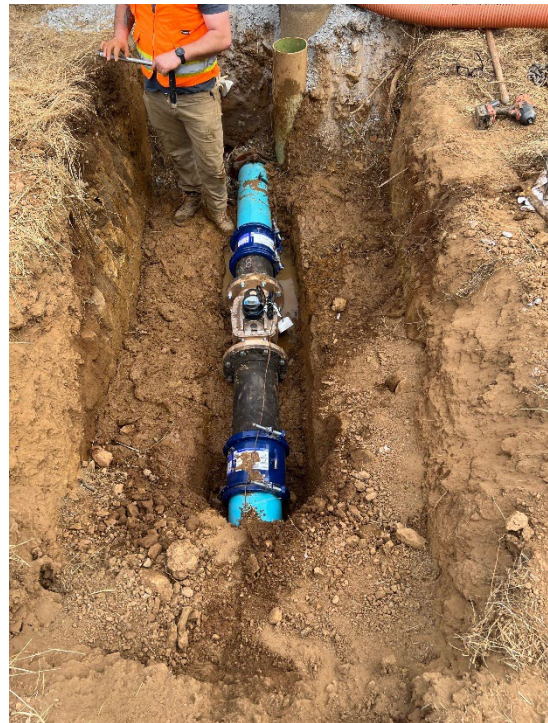
Pilot Hill Master Meter Install – 29 Labor Hours | Service Trucks, Dump, Excavator, Vac Trailer
