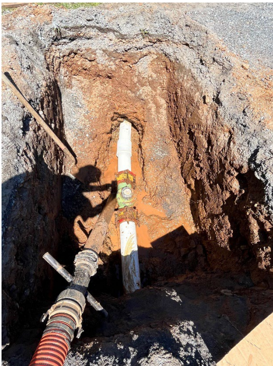
Master Meter Installation (Cherry Acres and Marshall Road) – 57 Labor Hours | Utility Trucks, Excavator, Material, Vac Trailer
