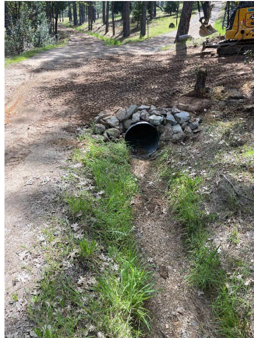
Culvert Repair – 16 Labor Hours | Excavator, Dump Truck, Service Truck
