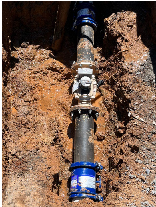
Master Meter Installation (Cherry Acres and Marshall Road) – 57 Labor Hours | Utility Trucks, Excavator, Material, Vac Trailer
