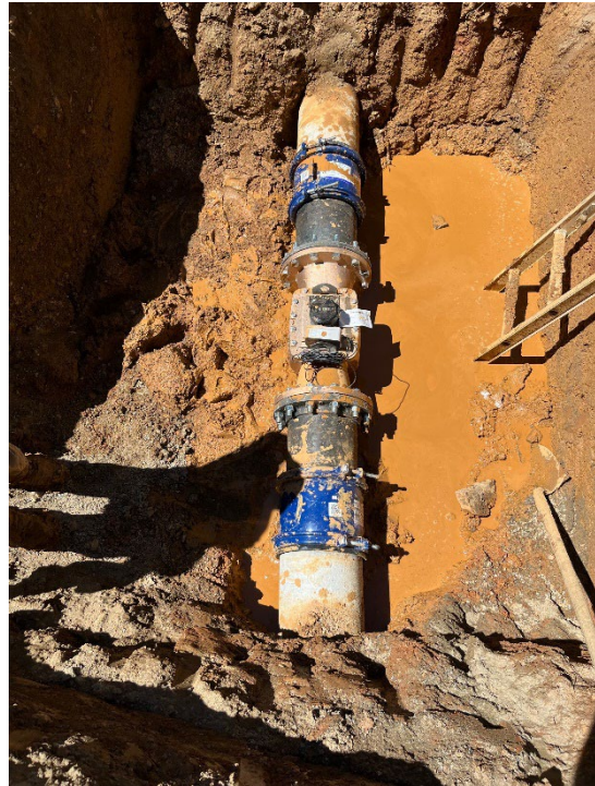
Master Meter Installation (Black Oak Mine Road) – 59 Labor Hours | Utility Trucks, Excavator, Material, Vac Trailer, Dump Trucks
