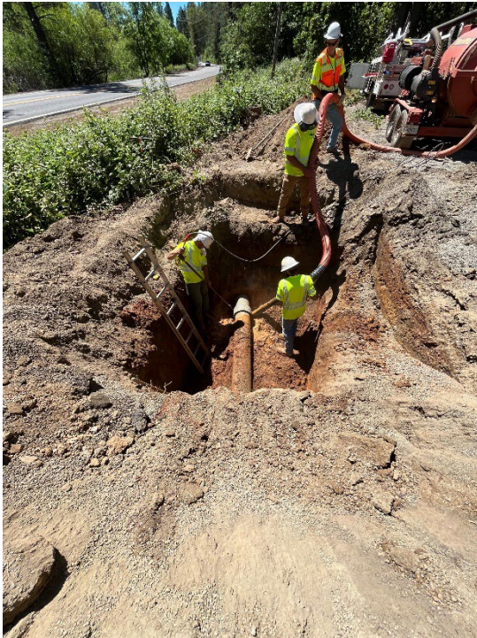
Master Meter Installation (Black Oak Mine Road) – 59 Labor Hours | Utility Trucks, Excavator, Material, Vac Trailer, Dump Trucks
