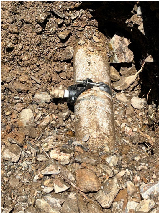
Saddle/Service Line Replacement – 24 Labor Hours | Excavator, Vac Trailer, Service Truck
