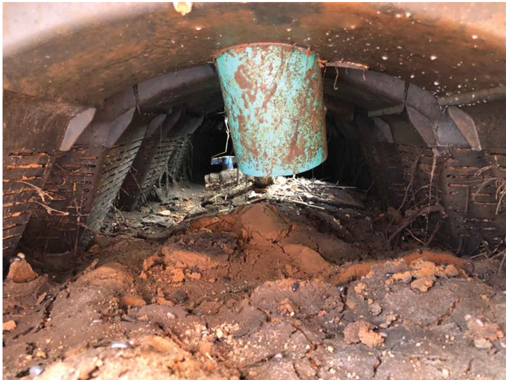
Photo No. 10 Looking into the northeast end of Field B, Row 2 infiltrator (looking to the southwest) (photo date 8/7/2020).
