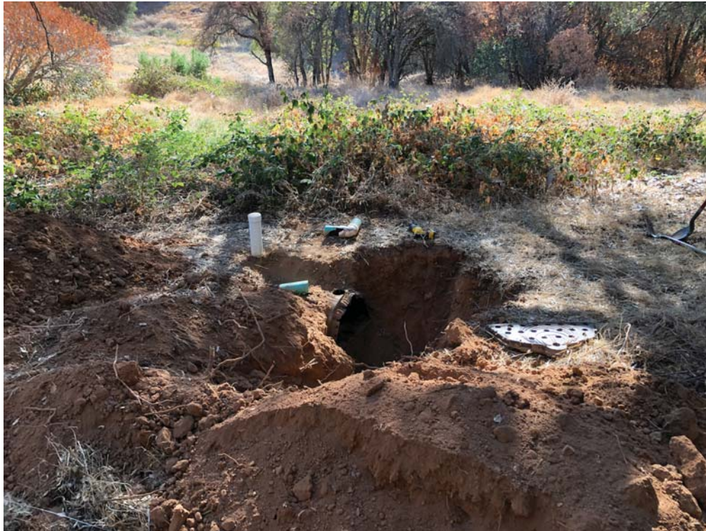
Photo No. 5 View looking east (downslope) at the southwestern portion of Field B and excavation LF2, exposing the end of an infiltrator (photo date 8/7/2020).
