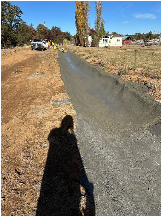
Canal Preparation/Lining – 180 Labor Hours | Service Trucks, Excavator, Hand Tools
