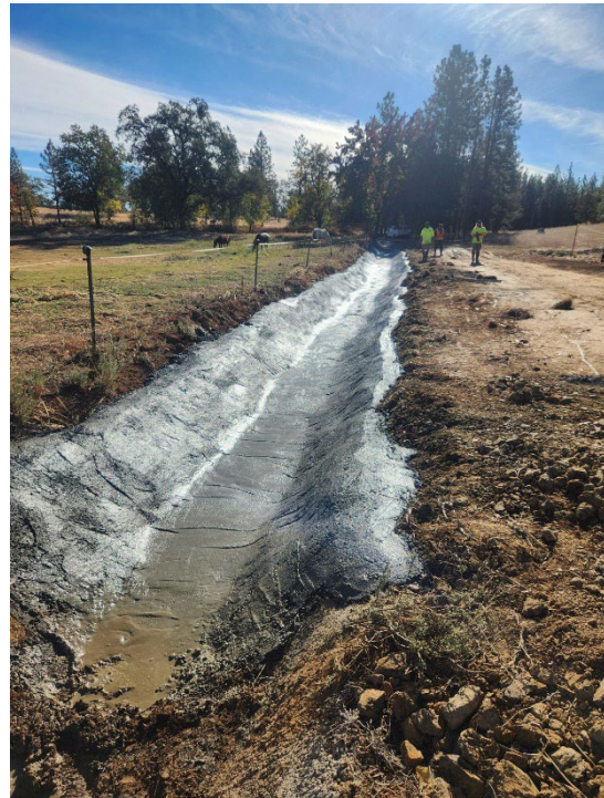
Canal Preparation/Lining – 180 Labor Hours | Service Trucks, Excavator, Hand Tools
