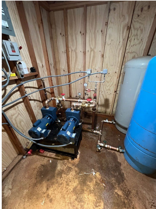
Reservoir Road Pump Station Rehabilitation – Control Panel, Pump and Plumbing Replacement
