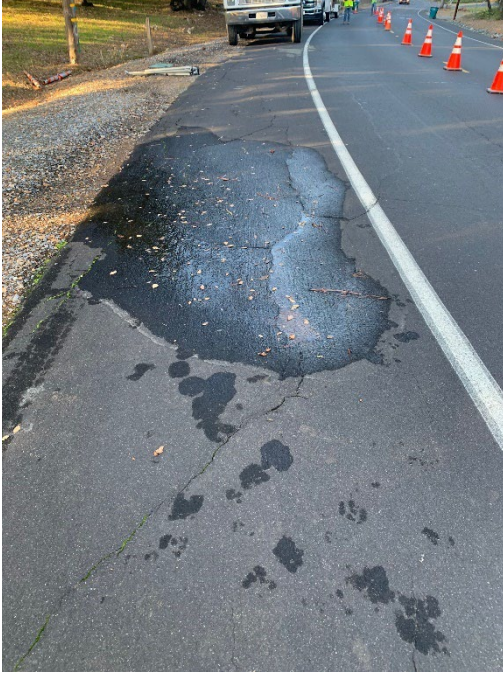
Main Break Repair – 27 Labor Hours | Dump Truck, Vac Trailer, Service Trucks, Hand Tools
