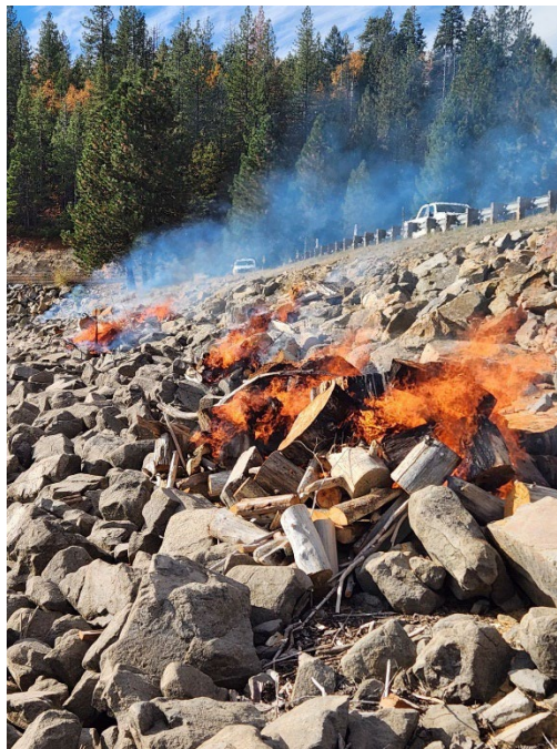
Vegetation Clearing Task – Debris Removal from Mark Edson Dam
