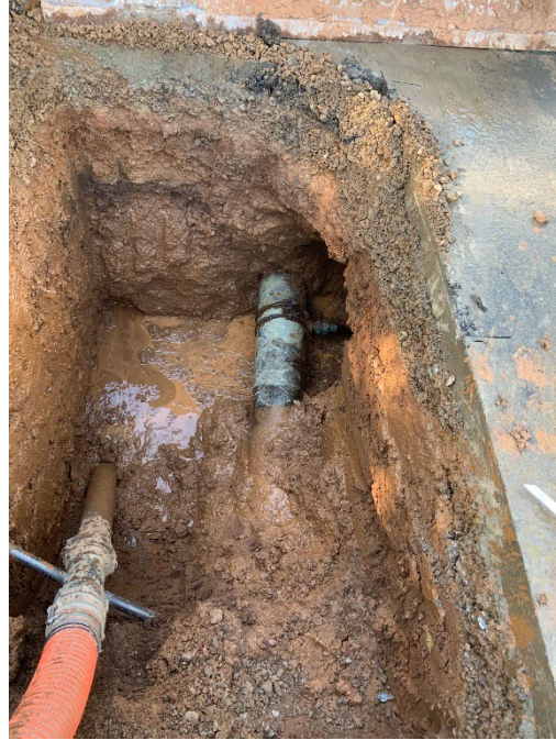
Main Break Repair – 27 Labor Hours | Dump Truck, Vac Trailer, Service Trucks, Hand Tools
