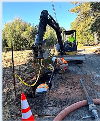
Meadowbrook Line Break Repair
