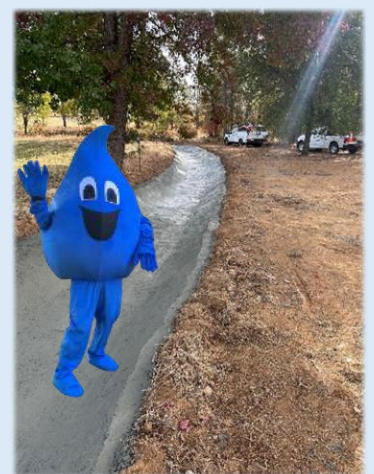
Canal Lining Project
