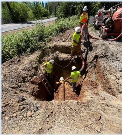
Master Meter Installation
